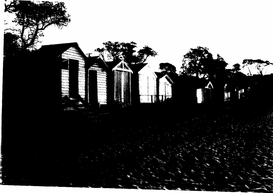
There are over 500 beach structures on the Shire's beaches, some more significant than others and a building type which demands more specialised study to reveal the historical associations behind each seemingly similar structure. This group on Town Hall Beach shows the traditional small gabled and weatherboard structures, with centred ledge & Braced doors, which proliferated on beaches after 1900 but existed in a more rustic form from the 1860s.
